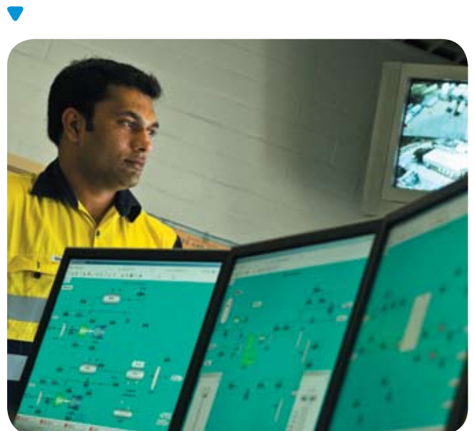
Air Liquide WA Graduate Process Engineer Raj Jadhav in the control room at Kwinana, Western Australia.
