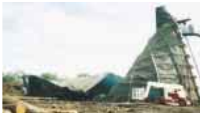
Demolition of the mill burner at Yarloop.
