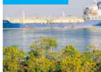
LPG ship tanker unloading gas at Kleenheat's Channel Island facility in Darwin, Northern Territory.
