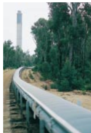
Above The conveyor belt delivering coal from Wesfarmers Coal's Premier mine to Western Power's new Collie power station, near Collie in Western Australia.
