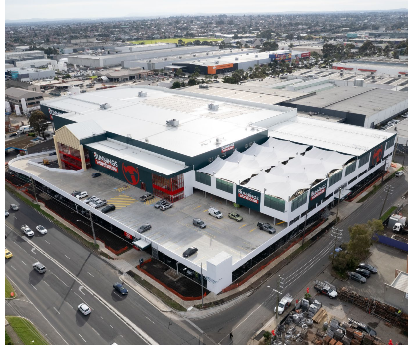
Preston Warehouse, opened July 2023
