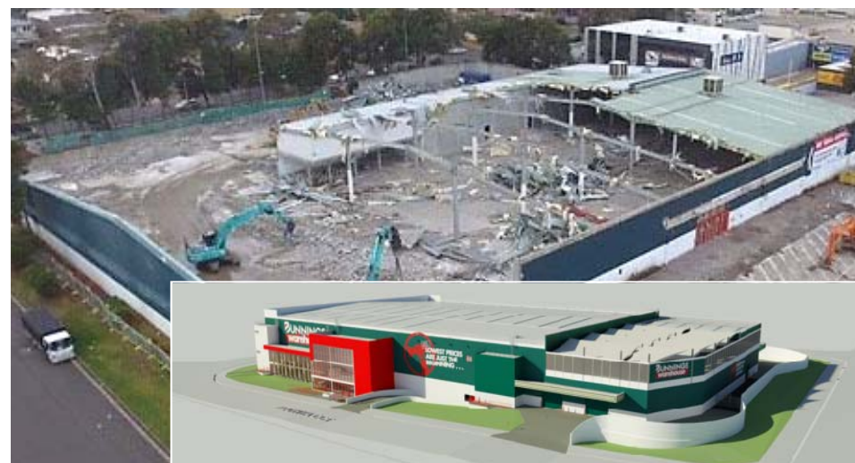
Caringbah, NSW store demolition & proposed new store
